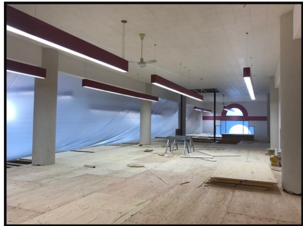
View from the south end of the mezzanine
